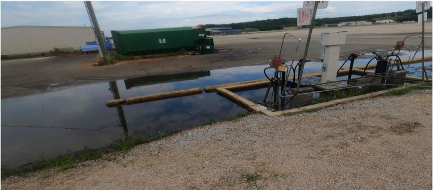
FUEL FARM C STANDING WATER
