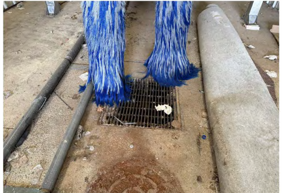
12> Inlet drain in wash rack area
