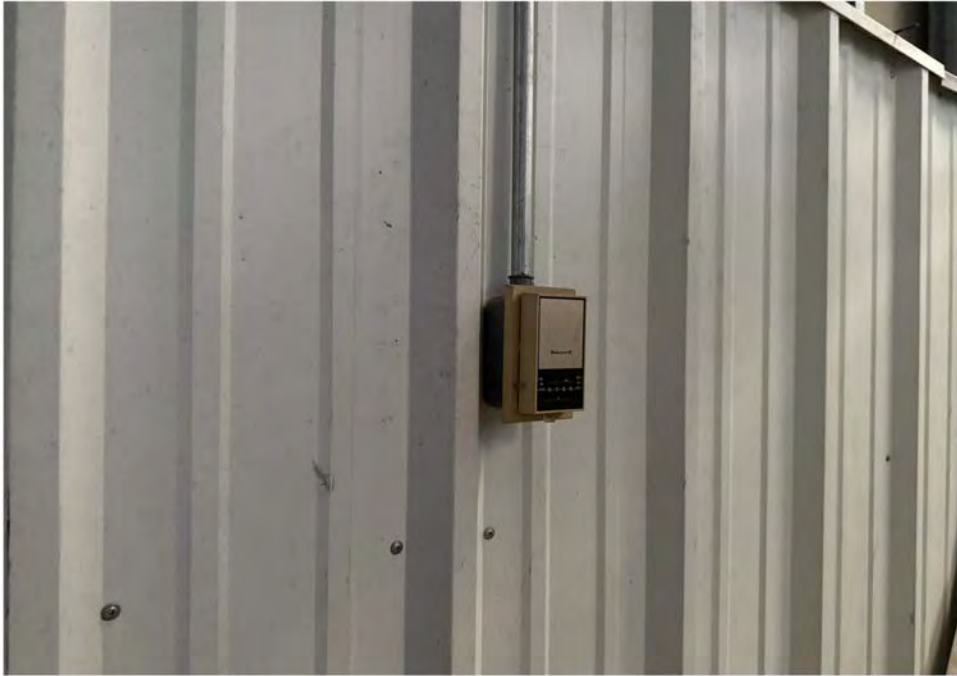
13> Mercury-containing thermostat in storage area between wash and service bays
