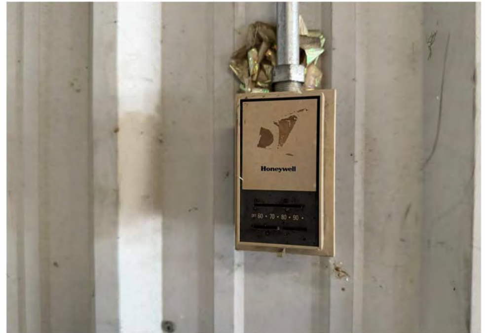
8> Mercury-containing thermostat in service bay
