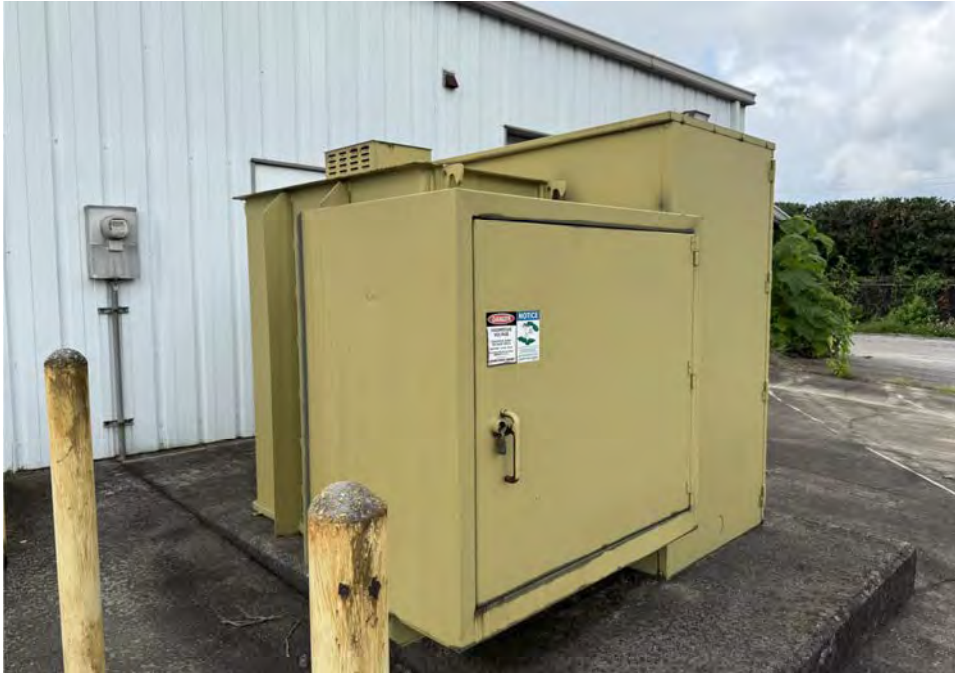
1> Transformer on north side of building
