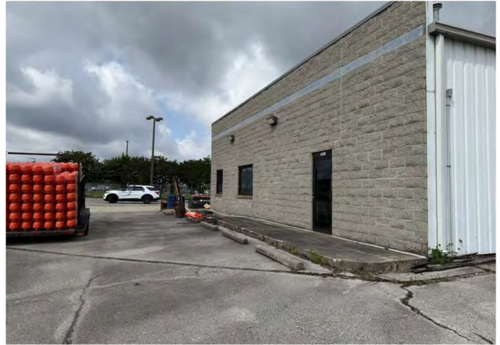
34&gt; Looking south along east side of building
