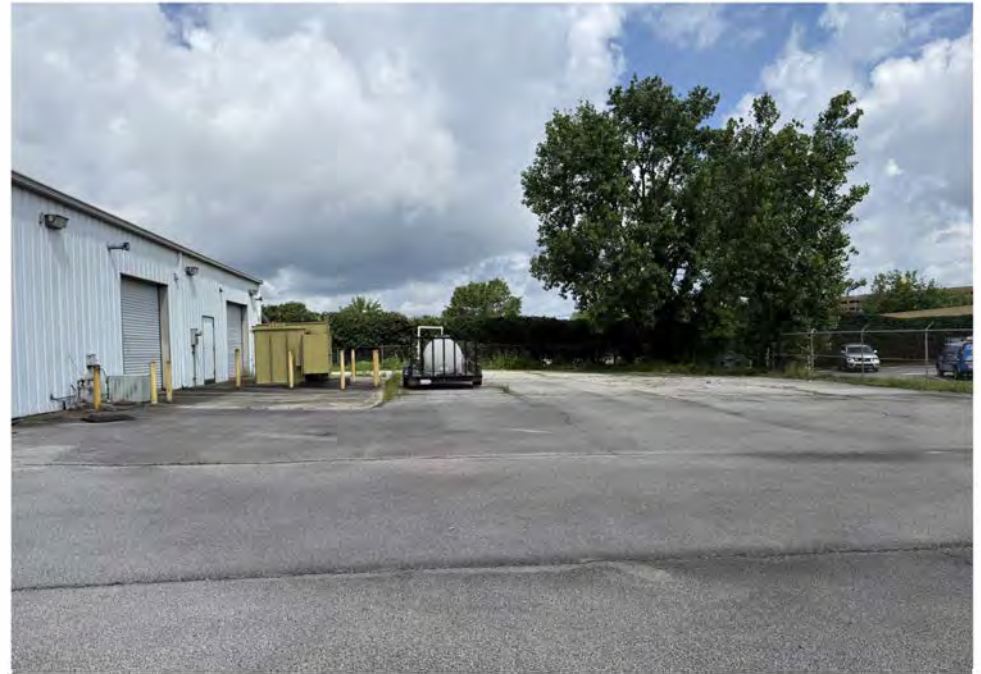
32> Looking west along north side of building
