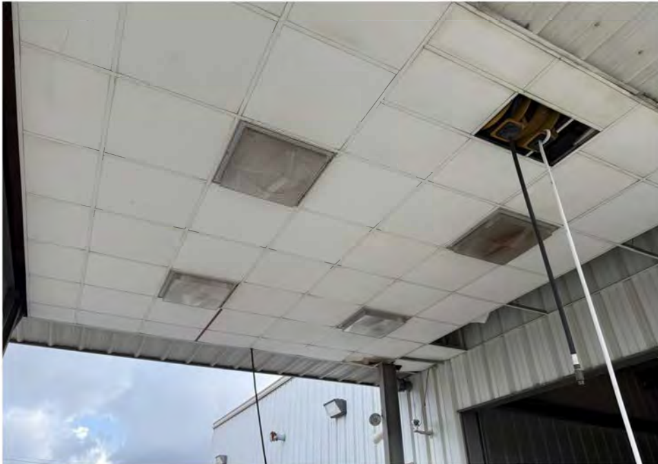
19> Ceiling area of wash bay lean-to
