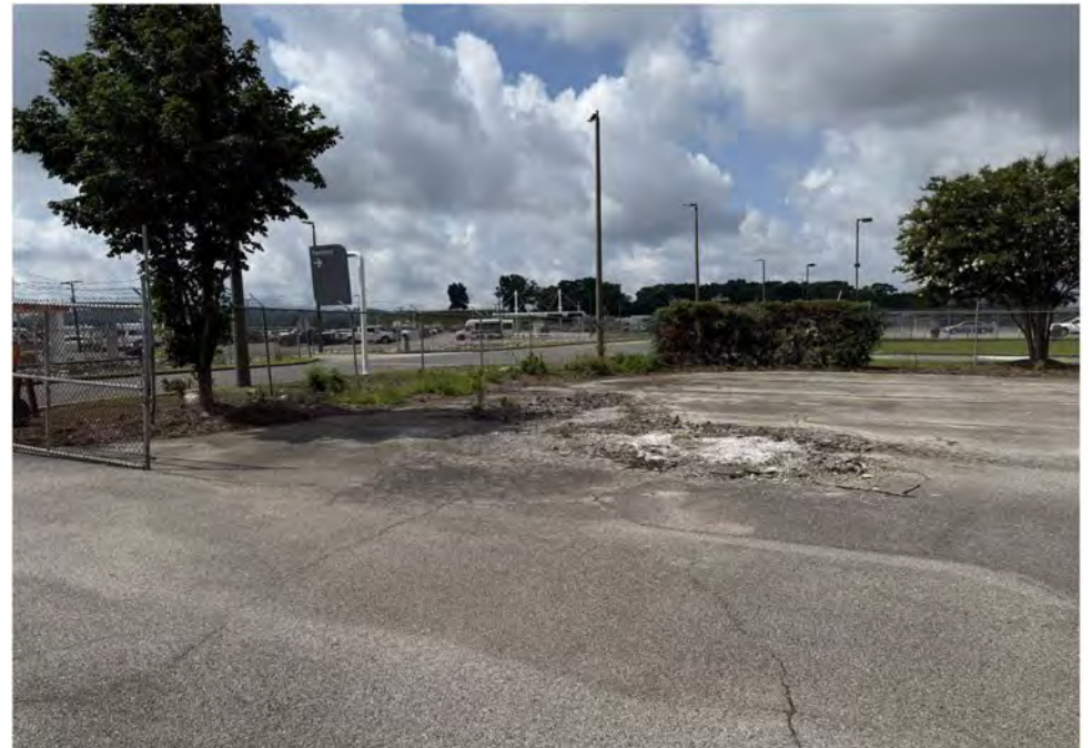
28> East side gate and entrance
