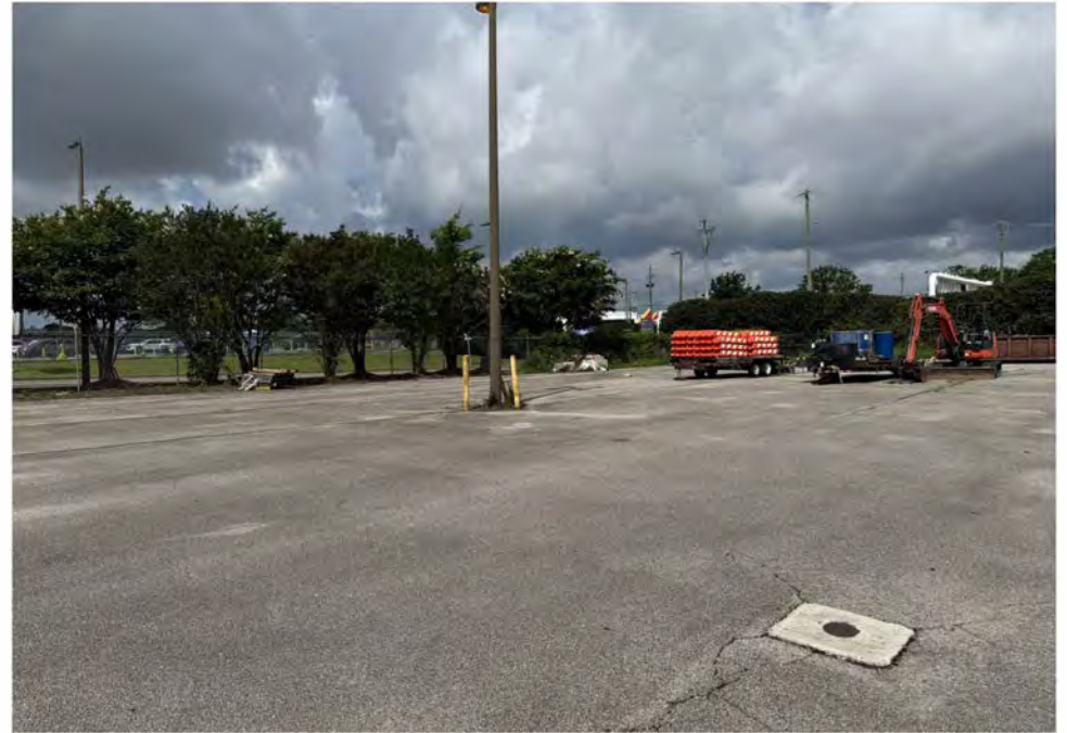
26> Looking south across pavement to SW corner
